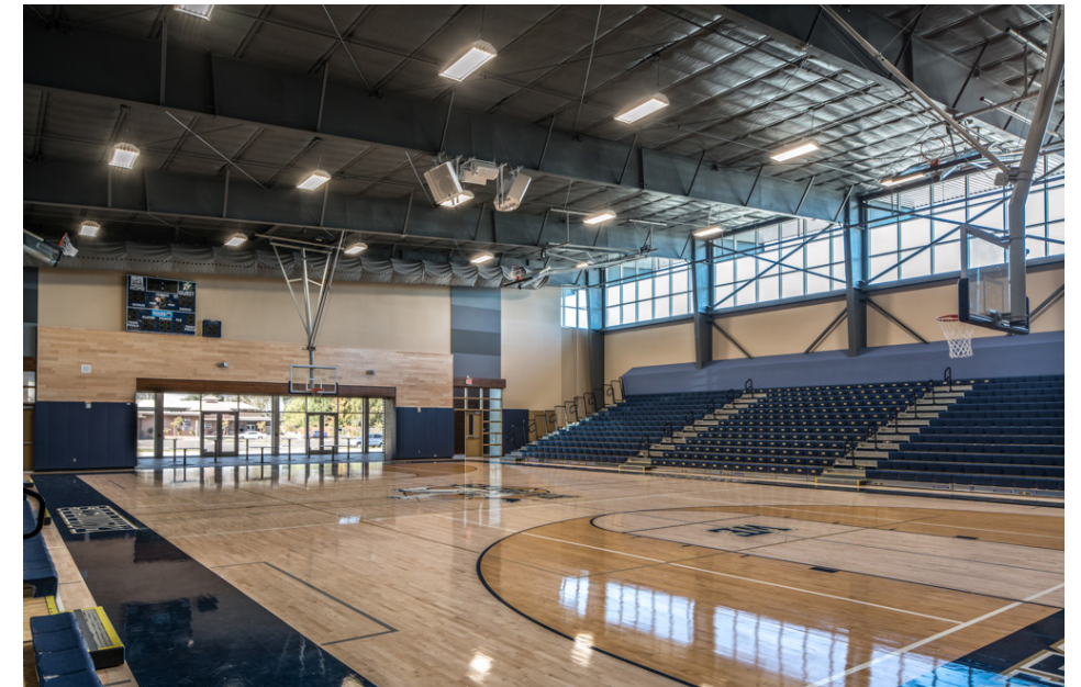
A distinct, inclining flat roof caps the gymnasium and allows for clerestory windows along the north side of the building to provide natural illumination.
